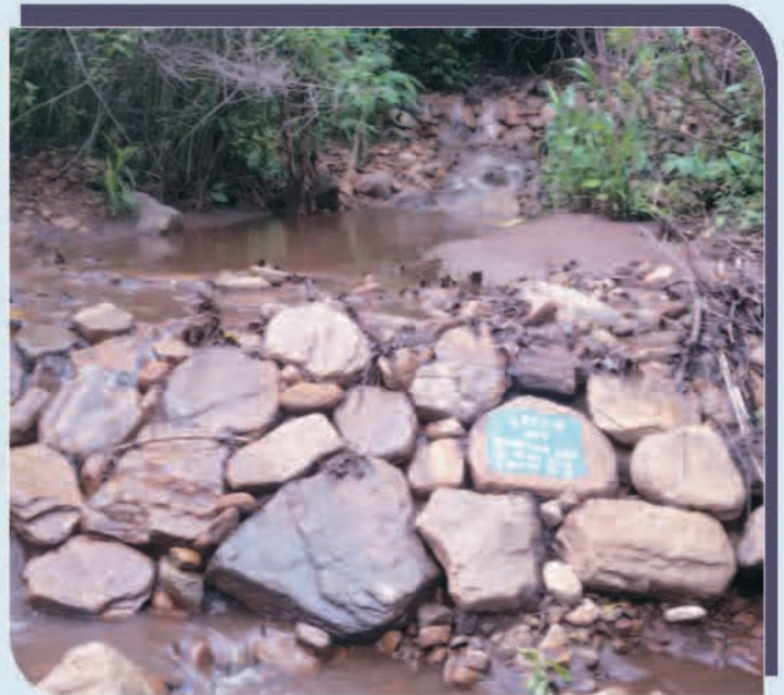
SMC work at Bandaka AJY VSS of Kotagarh FMU, showing the siltation and moisture conservation during monsoon.
