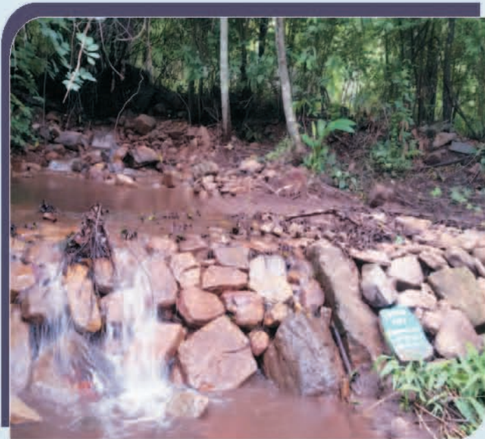
SMC work at Bandaka AJY VSS of Kotagarh FMU, showing the siltation and moisture conservation.
