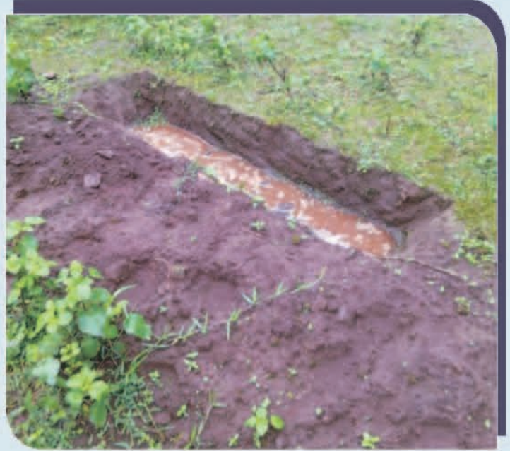
Staggered Trench at Kadgabali AJY VSS of Simonbadi FMU photo taken on 25/07/2017
