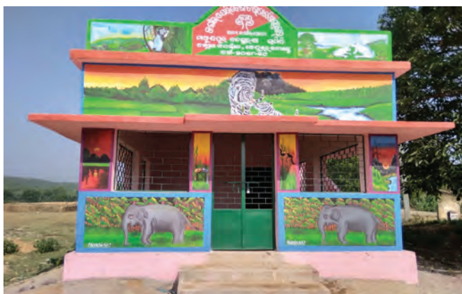
VSS Building at Makundpur VSS under Keonjhar Division
