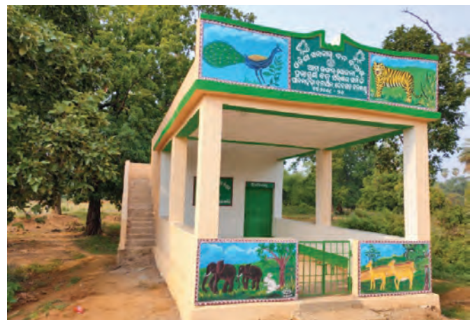
Building of Pravasuni VSS, Deogarh Division
