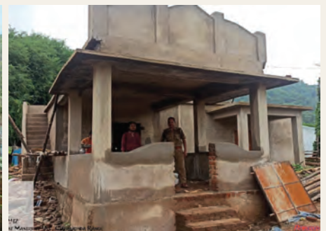
VSS Building of Sahid Lakhman Naik VSS is under construction
