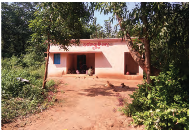
Anganawadi Center constructed under convergence with WoCD at Gauranga VSS, Angul Division
