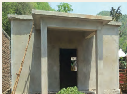
Community Hall under construction at Mantriput through GP Development Fund
