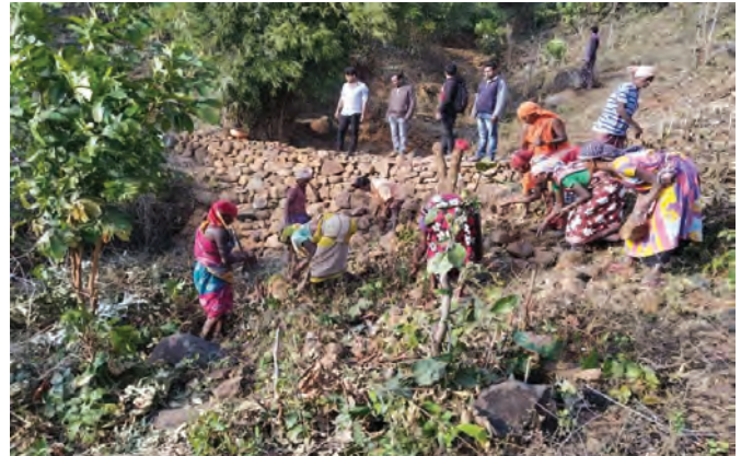
SMC Work at Mundinucha VSS, Keonjhar(WL) Division
