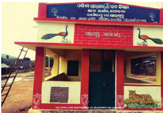
VSS Office cum Meeting Hall at Kilukumpa VSS, Phulbani Division
