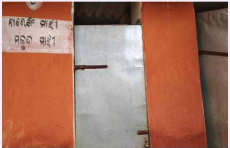
Sanitary Toilets constructed through Swachh Bharat Mission
