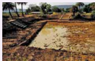
EPA in Khajuribahal VSS under Deogarh DMU
