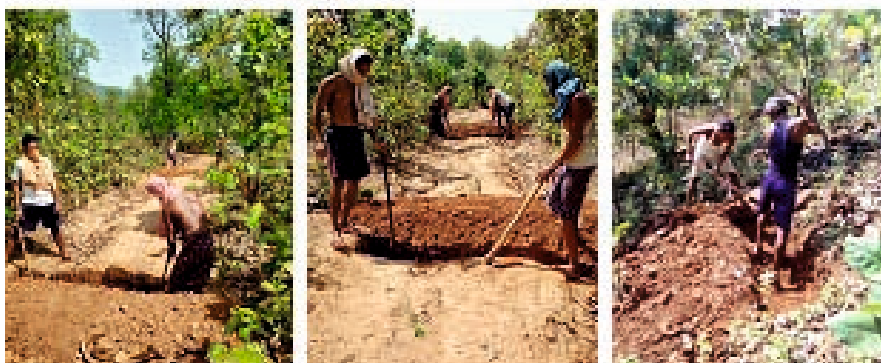
Staggered trenching in Asanpani & Bijadihi VSSs, Deogarh Division
