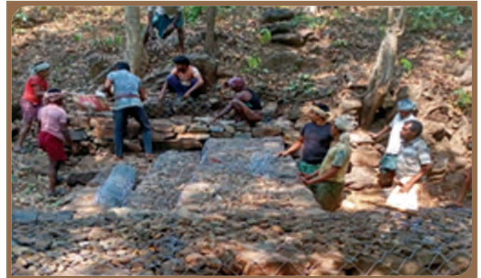
Wire Mesh LBCD at Badakhol VSS under Rairakhol Division
