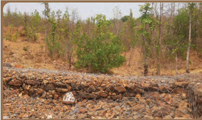
Wire Mesh LBCD at Medinipur VSS, Keonjhar Division
