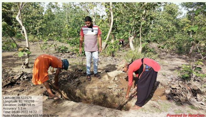
Renovation of staggered trench at Madkamiguda VSS, Malkangir Division
