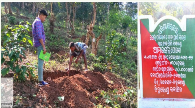
Renovation of Staggered Trench at Champajhola VSS, Malkangir Division
