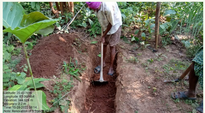
Renovation of staggered trench at Muribahal, Bolangir Division
