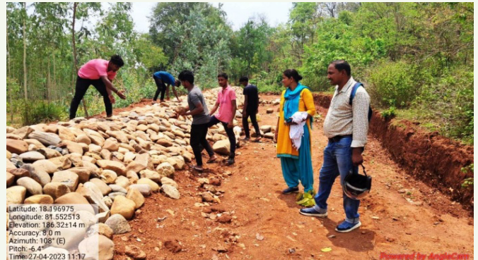
LBCD work at Tegadapali VSS, Malkangir Division
