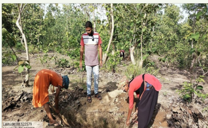
Renovation of staggered trench at Madkamiguda VSS, Malkangir Division
