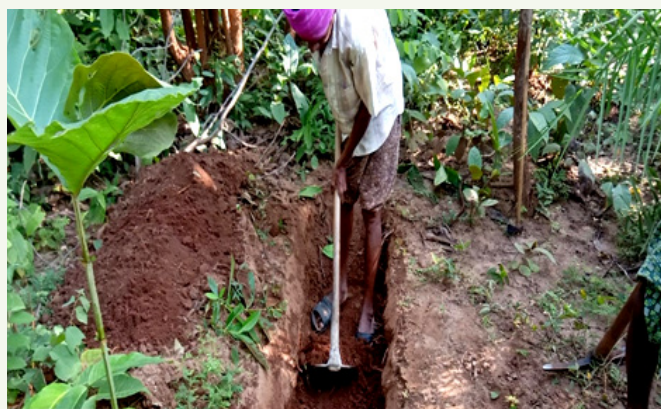
Renovation of staggered trench at Muribahal, Bolangir Division
