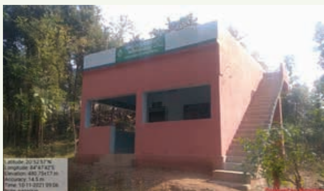
VSS office cum meeting hall at Tentuli VSS, Angul Division
