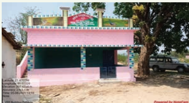
VSS building cum office at Petpura VSS, Deogarh Division
