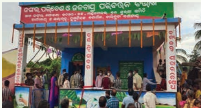
VSS building cum meeting hall at Mandalpadar VSS, Baliguda Division
