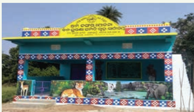
VSS office cum meeting hall at Nuasahi VSS, Phulbani Division
