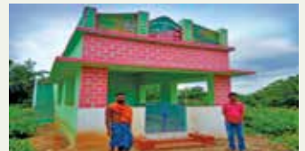
VSS building of Sangam VSS, Keonjhar WL DMU
