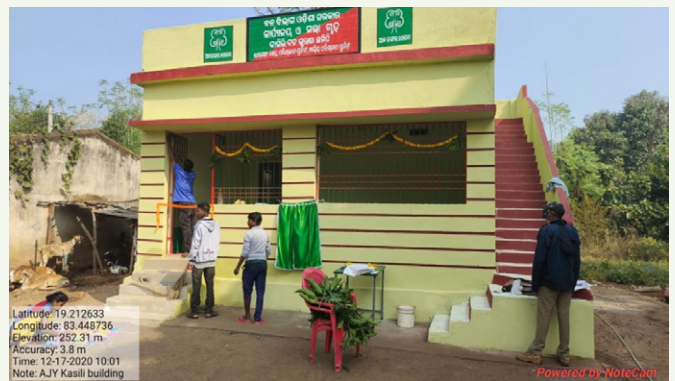
VSS Building-cum-IGA Facilitation Centre, Kasili VSS, Rayagada Division
