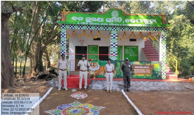
VSS Building-cum-IGA Facilitation Centre at Dhepaguda VSS, Jeypore Division
