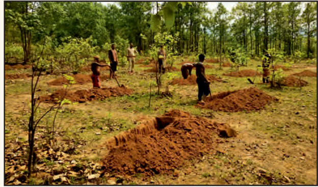
Staggered Trench at Kodiposha VSS of Keonjhar Division
