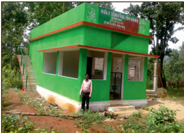
VSS Building of RANGADIHI VSS, KEONJHAR DMU
