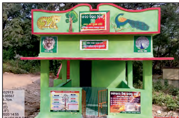
Office Building of Teda VSS, Koraput Division
