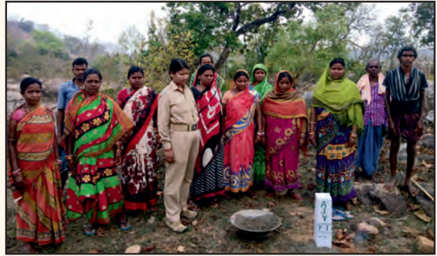
RCC pillar posting at Jharbeda VSS of Keonjhar Division
