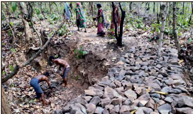
LBCD work at Sadangabahali VSS, Keonjhar Division
