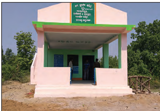
Office Building Balarampur VSS, Angul Division
