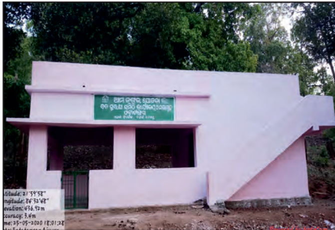
Office Building of Fatatangar VSS, Bonai Division
