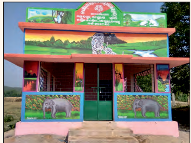
VSS Building of MUNDAPUR VSS OF KEONJHAR DMU
