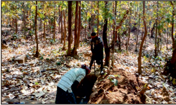
Staggered Trench at Khajuribani VSS, Keonjhar Division
