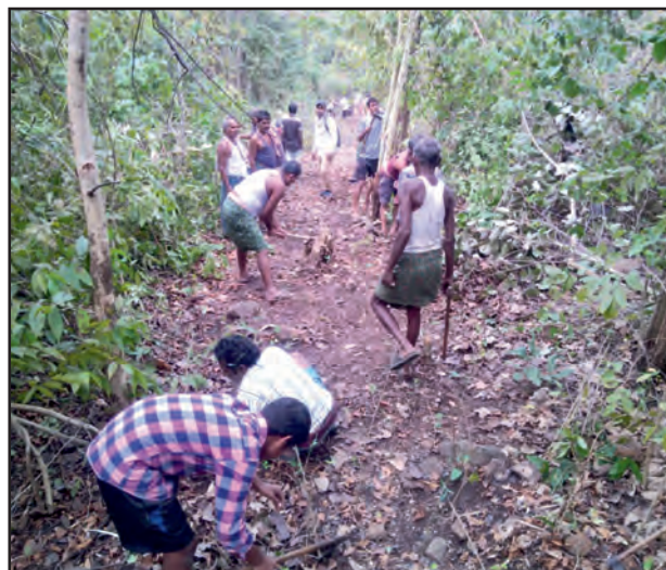
Fire line work at Karabira VSS, Angul Division
