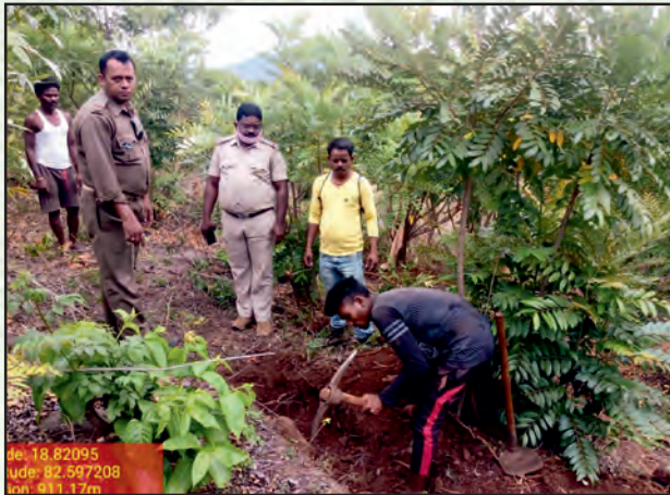
Staggered trench, Doudapadara VSS, Jeypore Division
