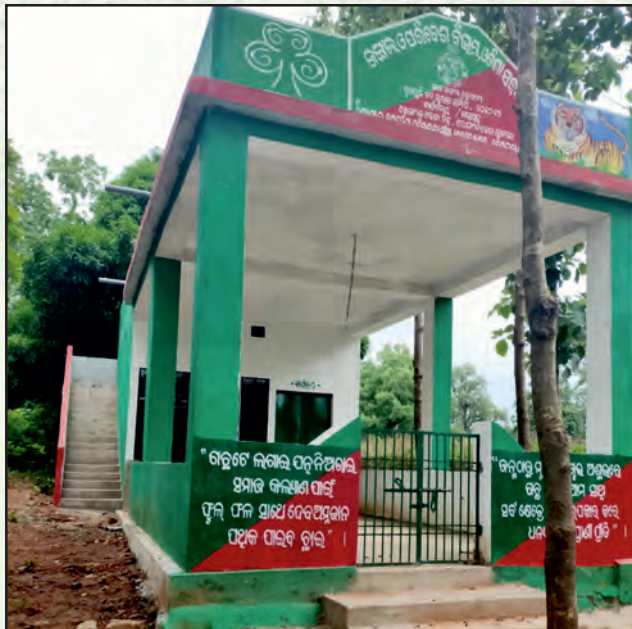
VSS building of Gujahuli VSS, Deogarh Division
