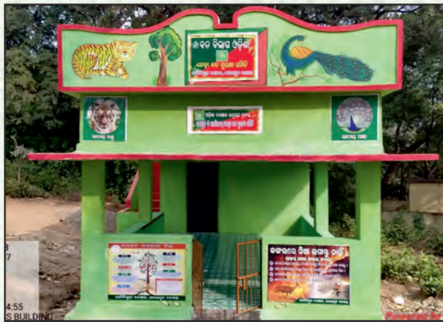
VSS building of Teda VSS, Koraput Division
