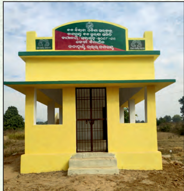
Bagmunda VSS building, Kalahandi-North Division
