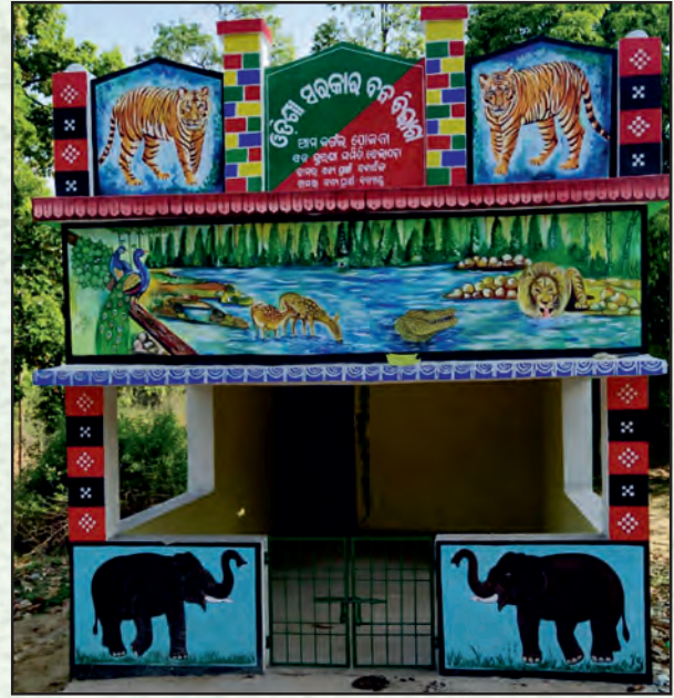
Belapada VSS building, Bamra WL Division
