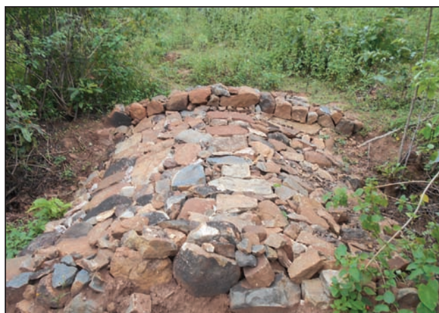
SMC works in Belaguda VSS of Laxmipur Range of Koraput Division
