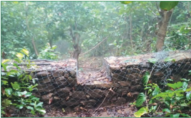
DLT work under Kairighati VSS
