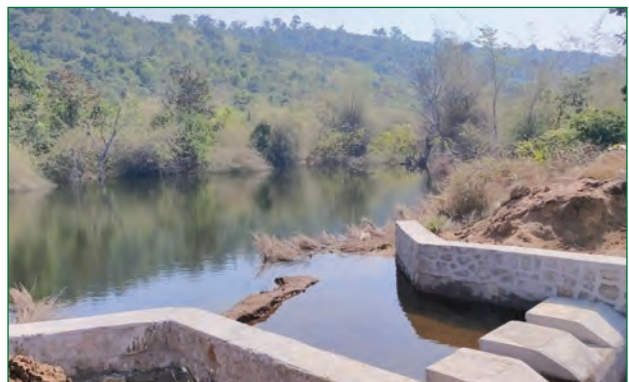
Check Dam created under Junani VSS
