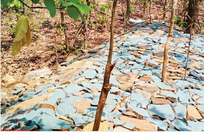
DLT Works in JFM at Purunapani VSS, Karanjia DMU
