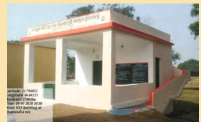
VSS Building-cum-IGA centre of Itamundia VSS
