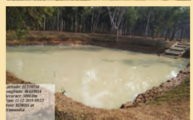
Progress of LBCD work in Itamundia VSS
