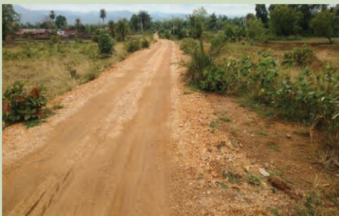
Kuchha road built in Gundisar VSS
