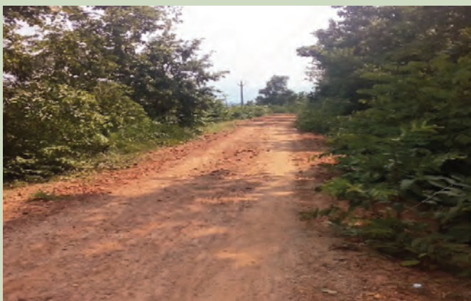
Kuchha road built in Berdabri VSS
