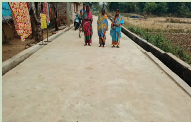
Concrete road built in Nuapada VSS
