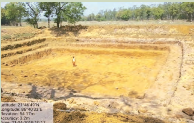
Progress of LBCD work of Hudisahi VSS Baripada
