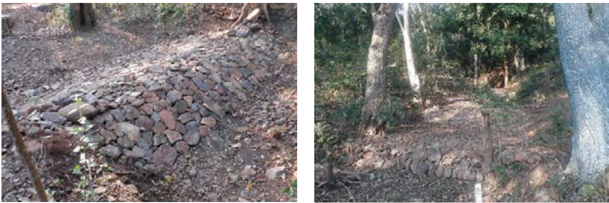
Check dams constructed
