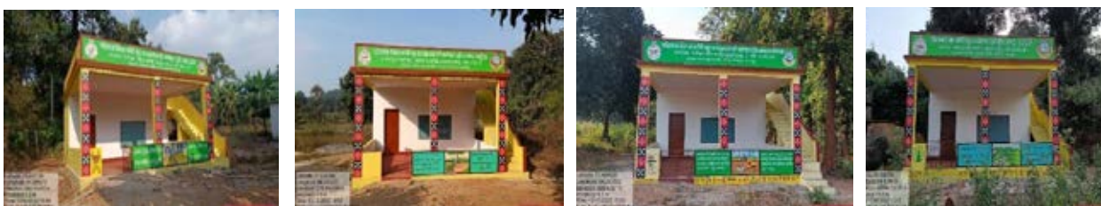
Completed VSS buildings
