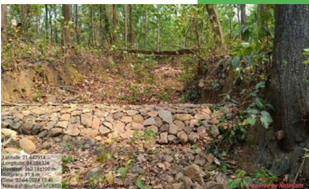
Check dam at Ghudiamba Nala 7
