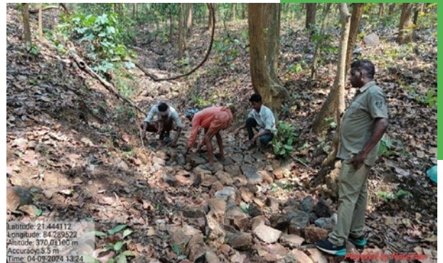
Check dam at Ghudiamba Nala 4
