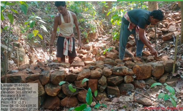
Check dam at Ghudiamba Nala 2
