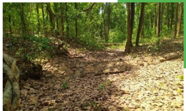
Check dam at Ghudiamba Nala 8
