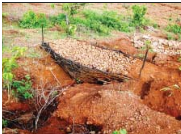
Brush wood check dams for gully plugs
